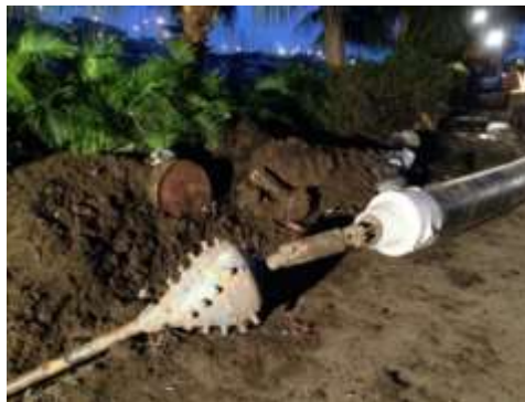
Gambar 3 Alat Back Reamer
