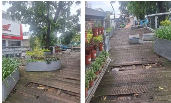
Figure 3. Poorly maintained park conditions, 2025. (Source: Personal)
