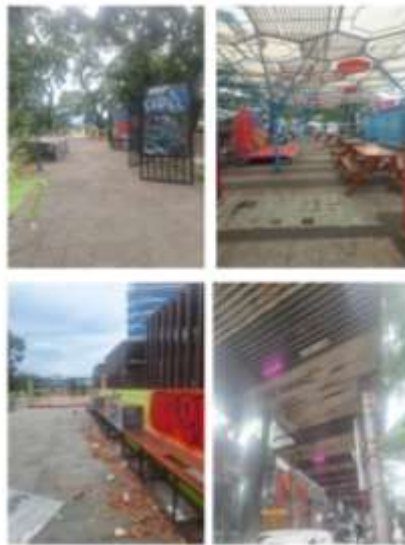
Figure 2. the condition of the Cihampelas terrace is not well maintained, 2025. (Source: Personal)
