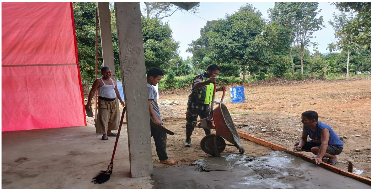
Gambar. 1 Proses Renovasi Lantai Balai Baca
